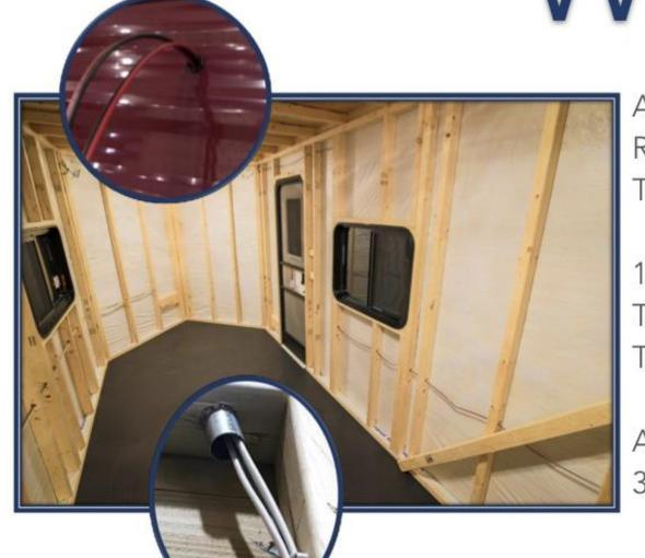
ALL WIRES RUN THROUGH RUBBER GROMMETS IN THE SHEET METAL
